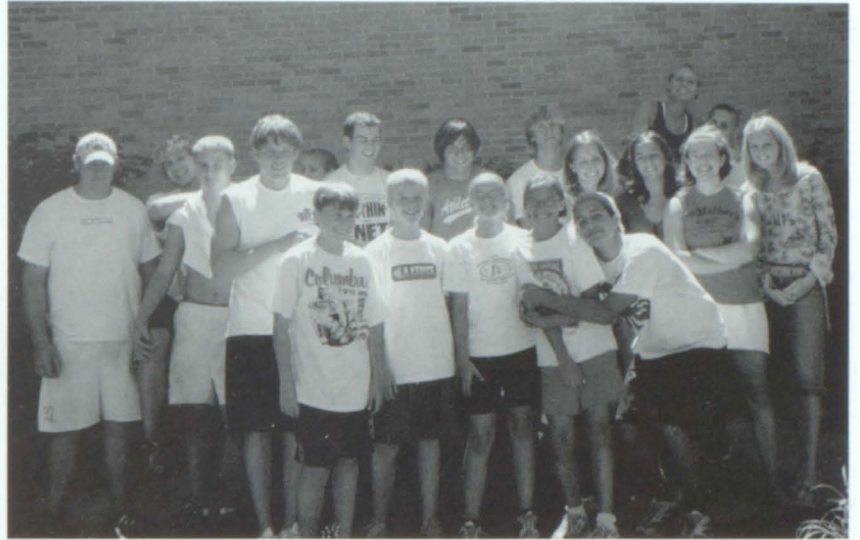
Some members of the courtyard reconstruction project take a break from their hard work.
